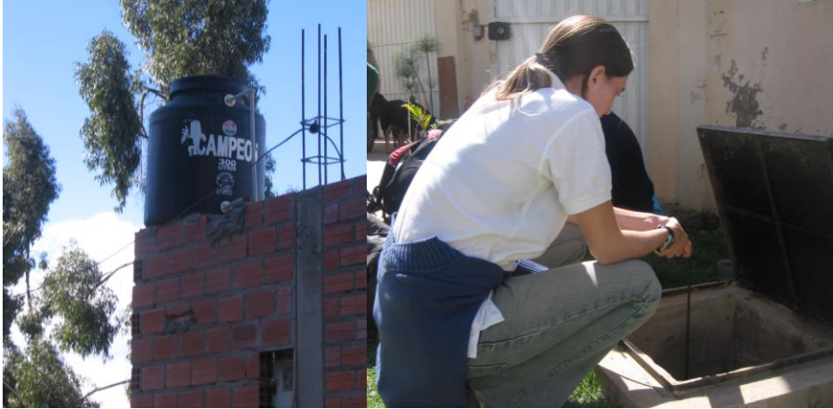
Figure 3: Elevated storage tank and cistern photos. a) Elevated water storage tank located on the roof of a home; b) Underground cistern located next to home near street.
